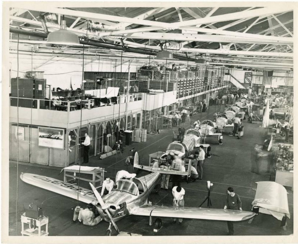
A line of Ercoupes at various stages of assembly at the ERCO factory in 1946. (Courtesy College Park Aviation Museum)
